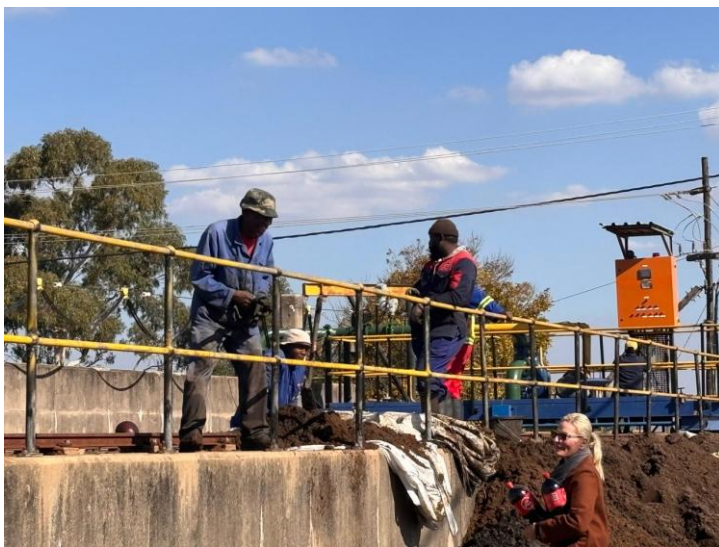
Phase 2 Filtration system at Bronkhorstspuit Water Treatment Plant change out of sand in the filter: Picture taken 15 May 2026.
