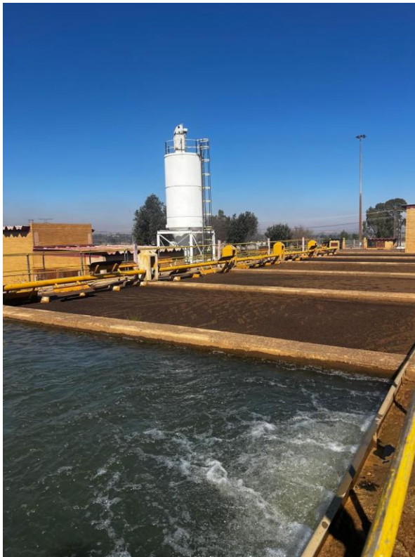
Phase 1 Filtration system at Bronkhorstspuit Water Treatment Plant: Picture taken 15 June 2026.
